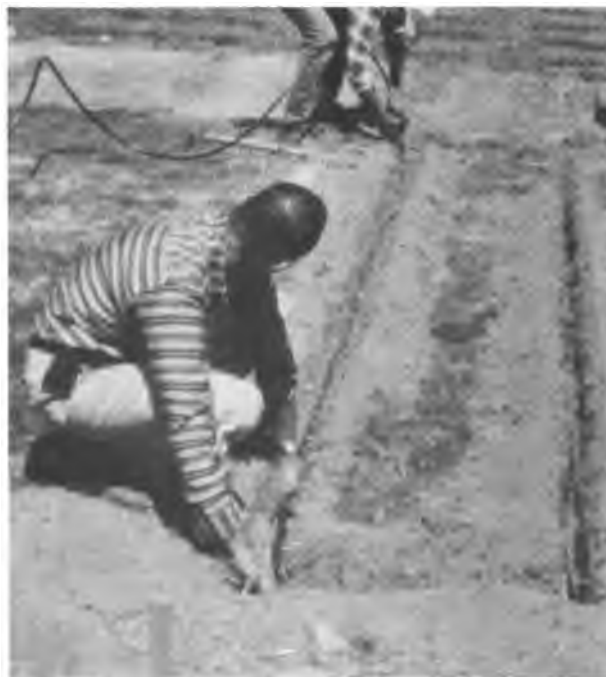
The expansion of cultivated areas implies a study of the more efficient methods to distribute and make the most of water resources, for irrigation purposes. An agricultural engineer, above, indicates how to bury the pipes for underground irrigation.
