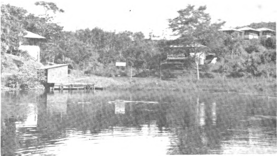
Dispensary, Store, and Three Laborers Cottages on Hill, Gasoline Shed and Dock at the Rubber Substation, Gatún Lake, Panama Canal Zone
