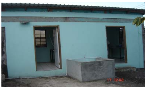
Newly established building site for the processing of Nelly's plantain chips
