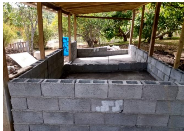
Figure 10: Composting shed post rehabilitation
