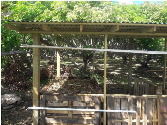
Figure 9: Composting shed pre rehabilitation
