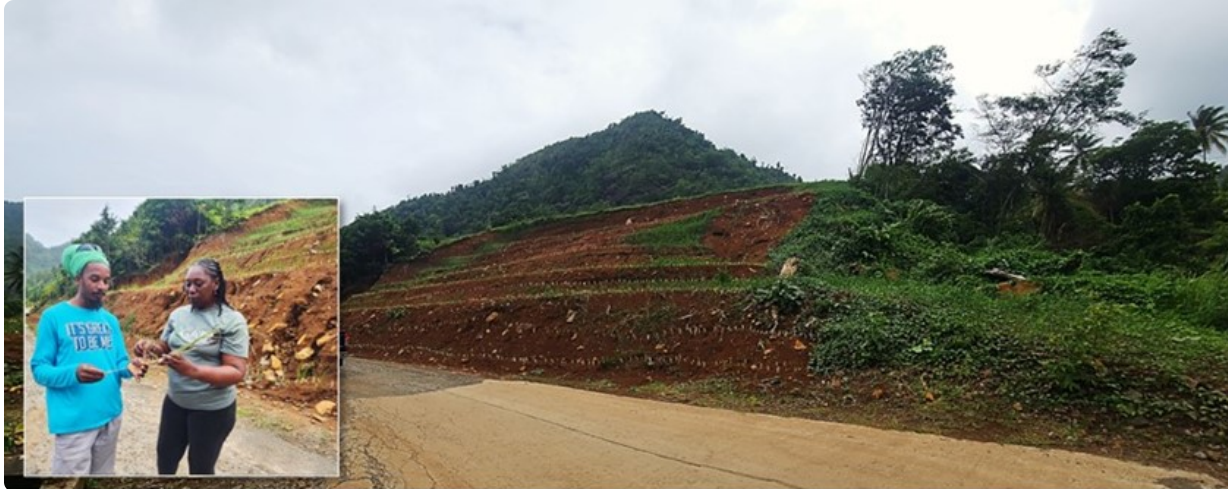
A site located in Petite Soufriere receiving the 'good grass' (vetiver) treatment, as described by project stakeholder, June Jackson from Antigua as she engages with project stakeholder, Elijah Charlemange from St. Lucia. (Photo: EbA project).
