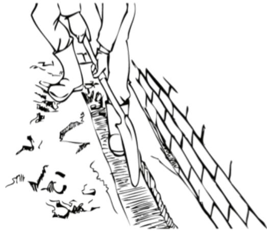
Dig trenches just outside of foundation wall and around sewer pipes and conduits in contact with the soil, before application of termiticide.
