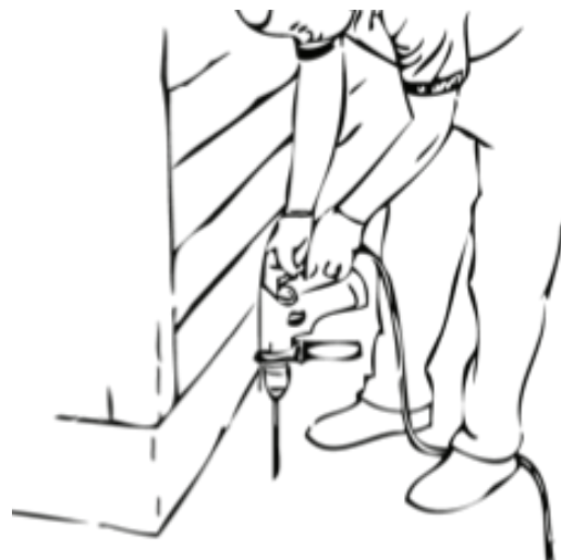
Application of termiticide.
