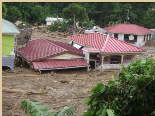
Landslide in Fond St. Jacques, Soufriere
