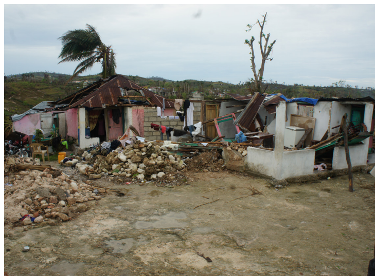
Devastation left by Hurricane Matthew in Haiti, 2016. (Source: IICA Haiti)
